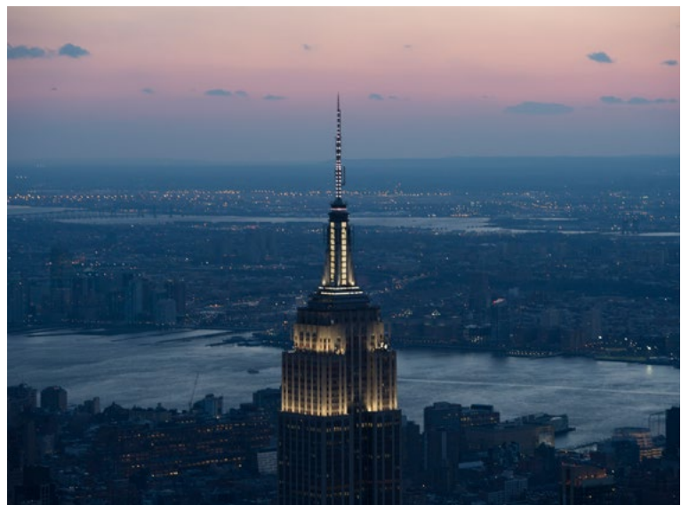
| Alfred R. Borden | Empire State Building, New York, NY | Client: Empire State Realty Trust | Alfred R. Borden, The Lighting Practice, Philadelphia and New York/USA | 2019 LIT Lifetime Achievement Award | Photo: Photographs courtesy of ESRT | © The LIT Design Awards™ |
